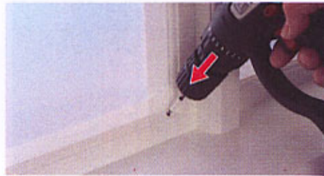
a2. Mark position as outlined in step 8 (over leaf). Drill Ø4mm hole to depth of 10mm
