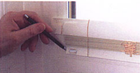
4. Using blind, mark positions for the cord grommet holes
