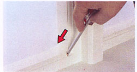
a3. Screw in brass inserts until flush with timber surface
