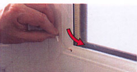
10. Push cord knot into hole, push fixing grommet into hole, aligning groove to cord
