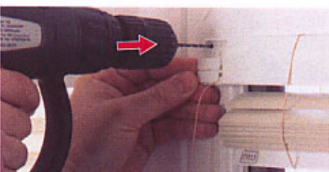
8. Drill Ø2.5mm holes 2 off on each side
