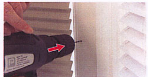
b3. Drill Ø2.5mm hole 1 off
